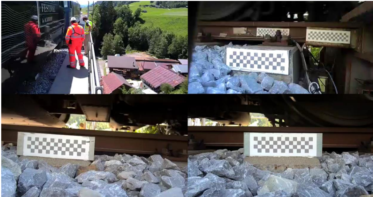
Views of the optical tracking cameras on one abutment of the railway bridge. The same system is replicated on the other side of the bridge.
