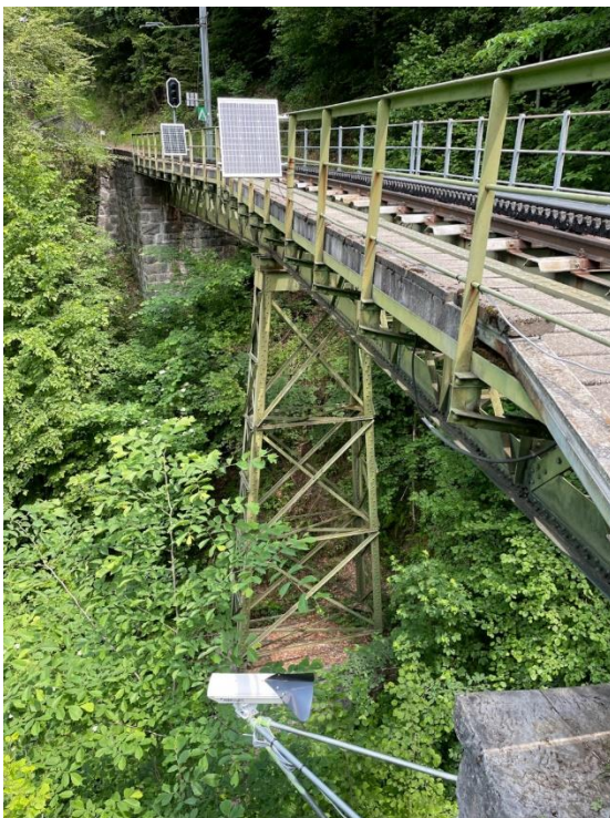
Left: View of the historical railway bridge with the solar power supply and one of the AIMsight autonomous optical monitoring systems. Right: View of the abutment wall monitored by the AIMsight system
