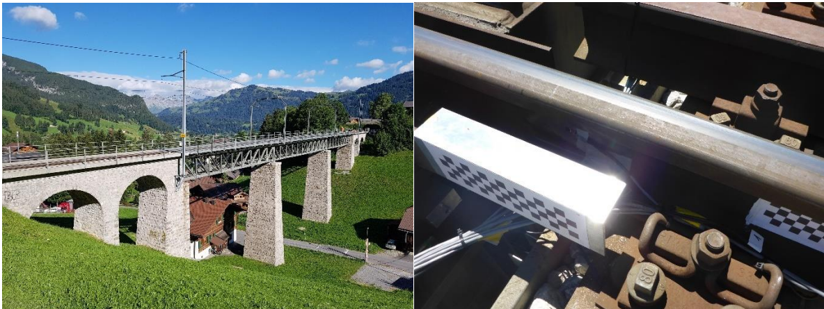
Left: View of the historical railway truss bridge. Right: Detail of the optical tracking pattern on the bridge and rail.
